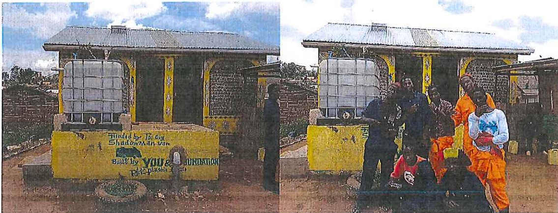
The Entire structure is made up of plastic bottles. It uses a composting system and recycles rain water.
