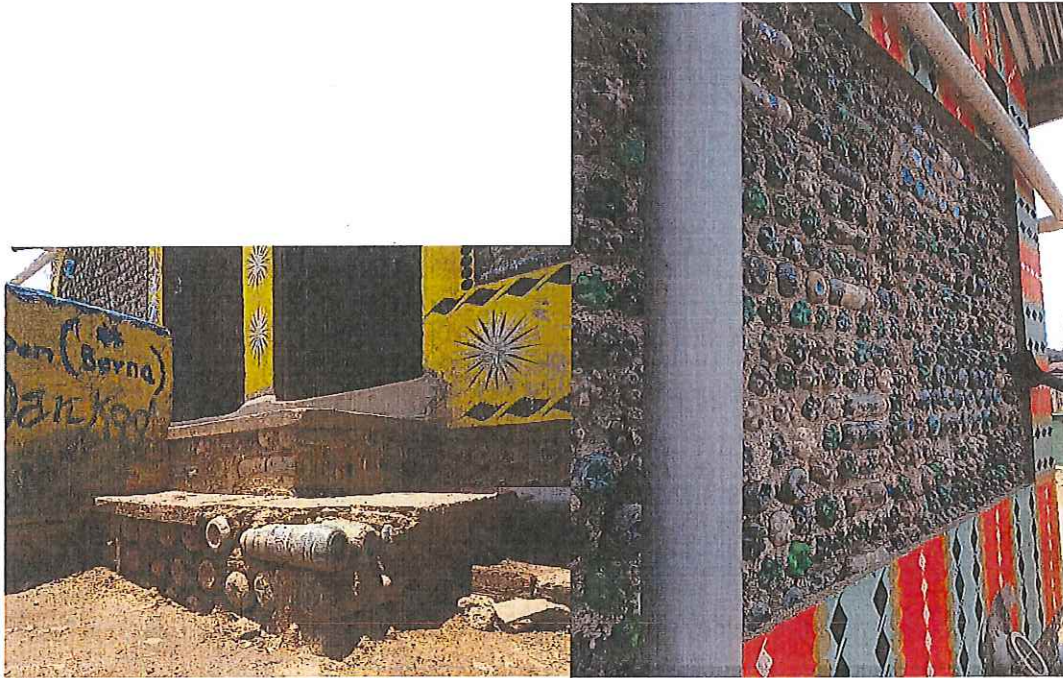
Pictures of the first structure in Kamokya. Even the foundation uses Eco Bricks
